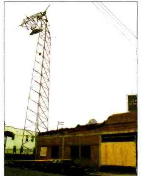
Winds over 100 mph obliterated MediaOne's microwave receive tower, knocking out retransmission of local broadcast stations.
